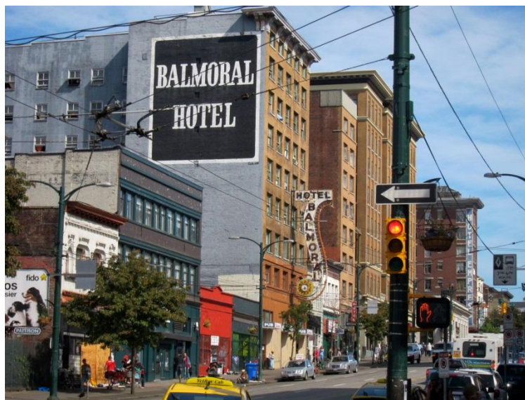
Fig. 2. The Balmoral Hotel is an emblematic example of an old, cheap and substandard hotel of Vancouver Downtown Eastside. The decline of SRO hotel rooms has only been partly replaced by residences operated by non-profit organizations. Photo B. Raoulx, 2013.
