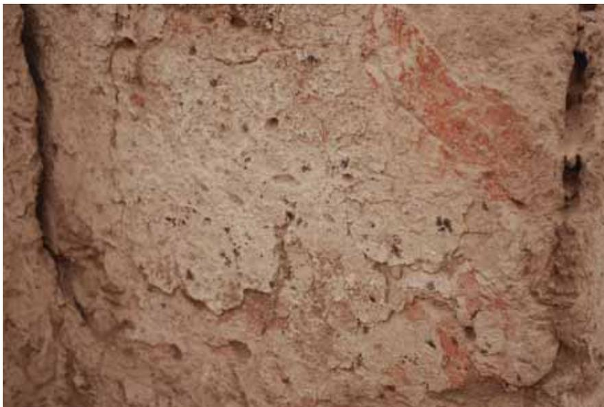
Fig. 13: the ochre coating of the doorway connecting Spaces No. 4 and No. 5.
